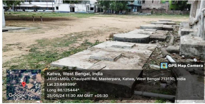
Waste water recycling through soak pit
