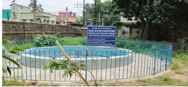
Rain water harvesting (ground water recharge circular shaped trough injection well)
